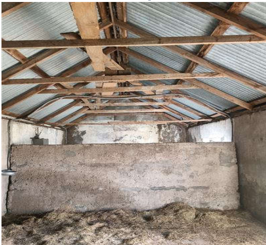
Plate 3-11 Stone Shed 3, interior
