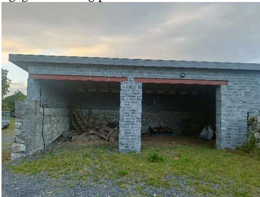
Plate 3-15 Shed, southern aspect
