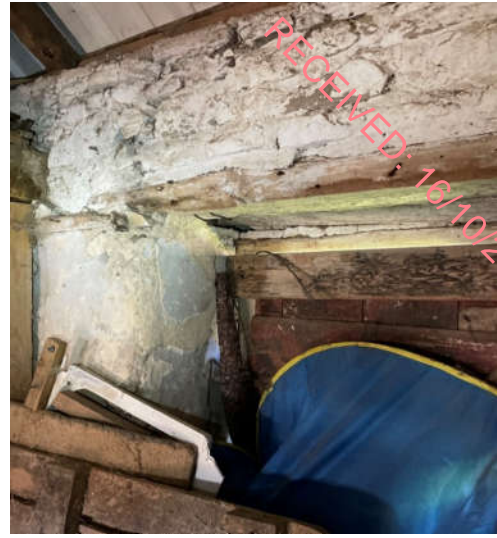
Plate 3-4 Stone Shed 1 interior
