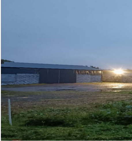
Plate 3-13 Large Shed, western aspect
